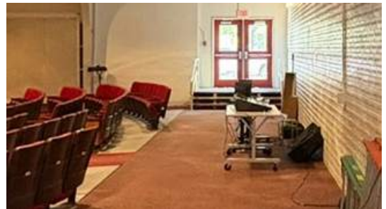
Exit doors with steps at back of house, operators in egress
