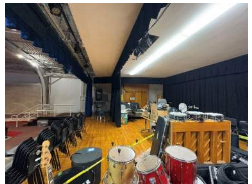
Existing ceiling overstage with draperies
