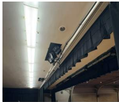
Sheetrock ceiling over stage
